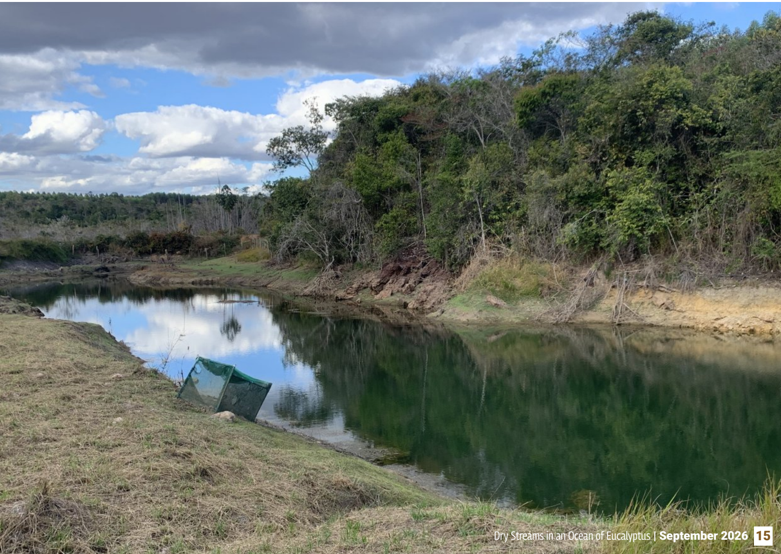
A small dam constructed to alleviate water scarcity for local residents. GFC
