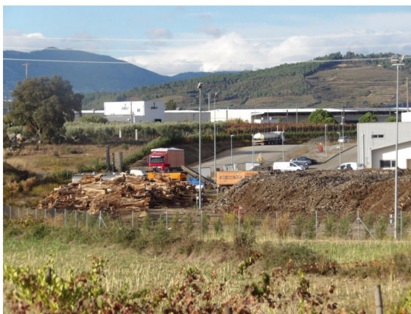
FIGURE 3 – Photo of biomass supplies at the plant
