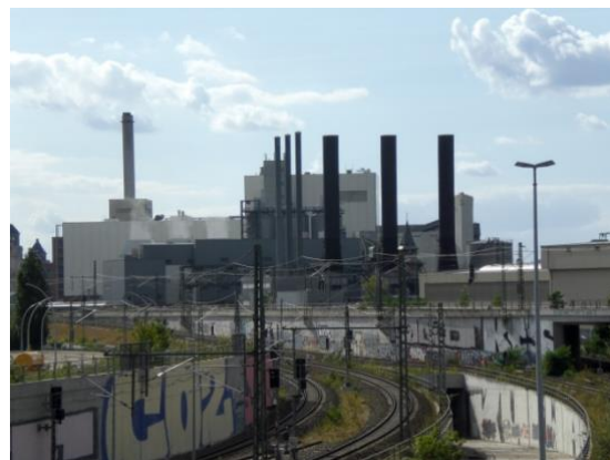
Moabit power and heat plant, Photo: Wikimedia
