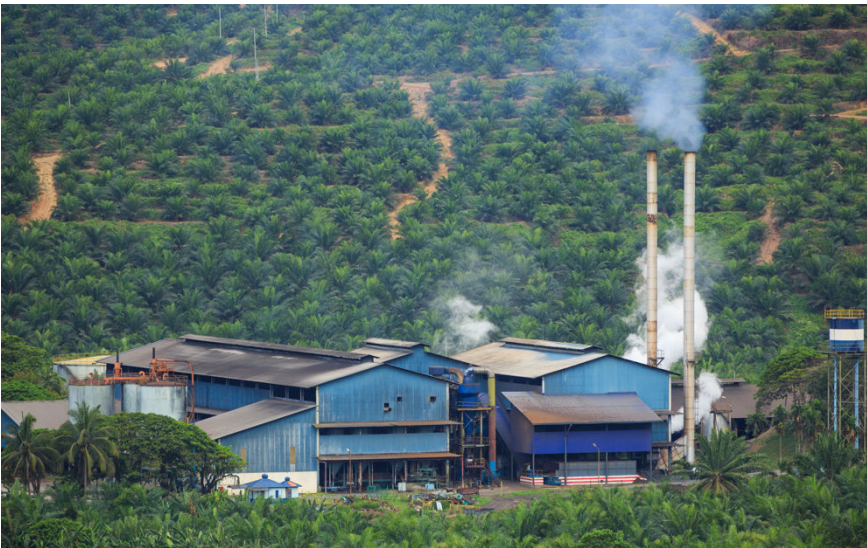
Palm oil mill in Malaysia. Credit: Uwe Aranas via Creative Commons
