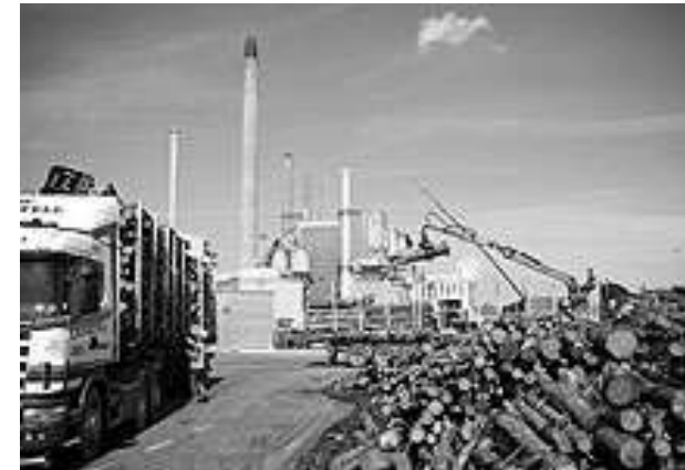
A biomass power station in Middlesbrough
