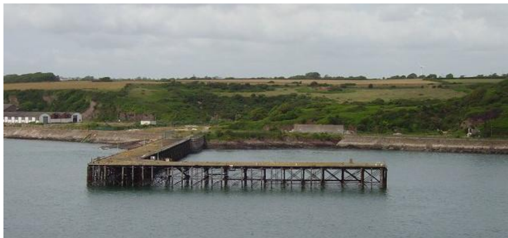
Site of the proposed biomass gasifier. Richard Webb, CC BY-SA 2.0
