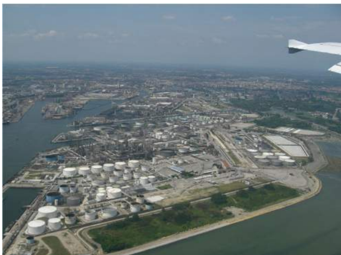
Eni's Porto Marghera refinery near Venice which has been converted to HVO production from palm oil, Source: panoramio.com/photo/40482299
