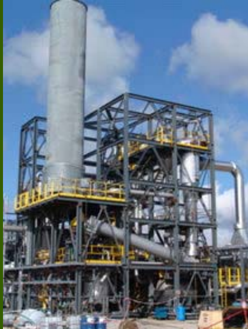
Dynamotive pyrolysis plant in Guelph, Ontario
