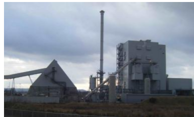
...To this? (Biomass plant: Steven's Croft, Scotland)
