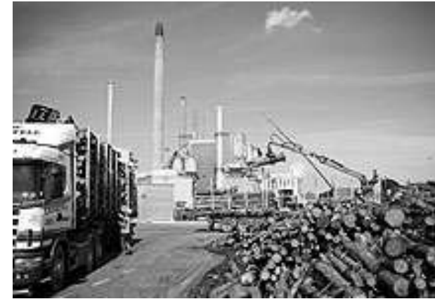
A biomass power station in Middlesbrough
